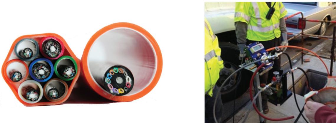
Figure 6. Air Blowing Light-weight Microcables Provides a Fast and Efficient Way of Increasing Transmission Capacity
