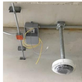
SDAN deployment examples from left to right: SDAN mounted in base of light pole, concealed behind wall face plate, installed on rack tray, deployed above ceiling to feed security camera, and hidden behind TV mount to deliver triple-play
