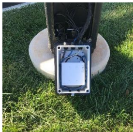
SDAN deployment examples from left to right: SDAN mounted in base of light pole, concealed behind wall face plate, installed on rack tray, deployed above ceiling to feed security camera, and hidden behind TV mount to deliver triple-play
