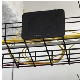
SDAN deployment examples from left to right: SDAN mounted in base of light pole, concealed behind wall face plate, installed on rack tray, deployed above ceiling to feed security camera, and hidden behind TV mount to deliver triple-play
