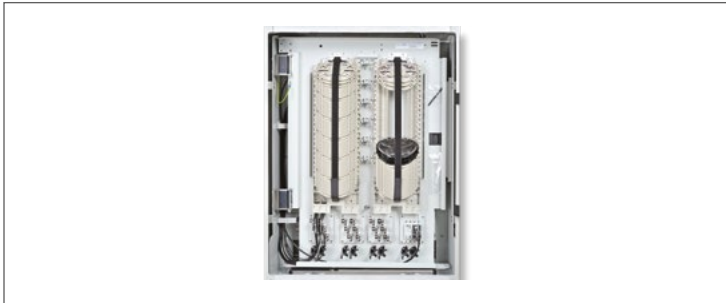
KVZ Street Cabinet Splice Area
