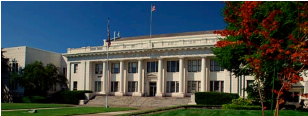
Douglas County Courthouse, Roseburg, Oregon. Source: Gary Halvorson, Oregon State Archives
