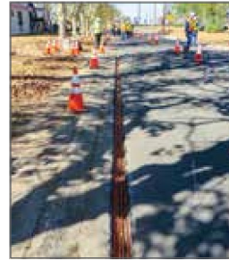
Step 1: Digging the micro trench
