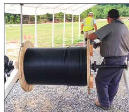
Figure 7. Payout of a 144-Fiber MiniXtend Cable
