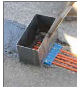
Figure 33. Microtrenching Method
