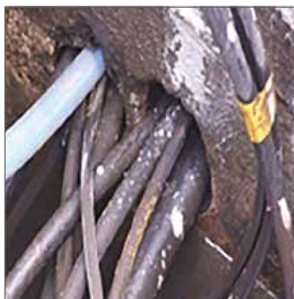
Figure 31. Congested Duct
