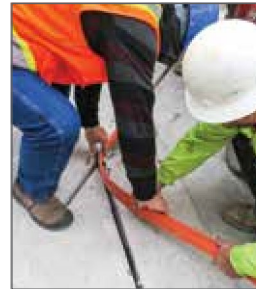
Step 2: Placing microduct in trench
