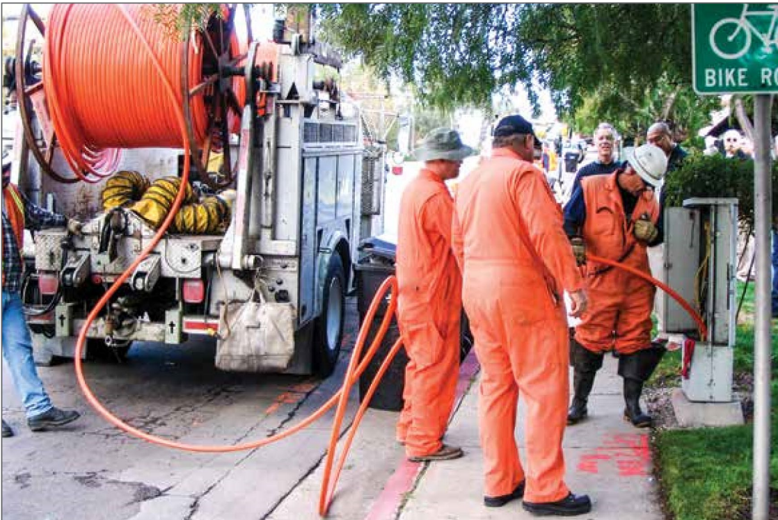
Figure 1. Microduct installation
