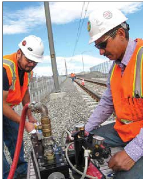
Figure 28. Micro Cable Blowing Installation
